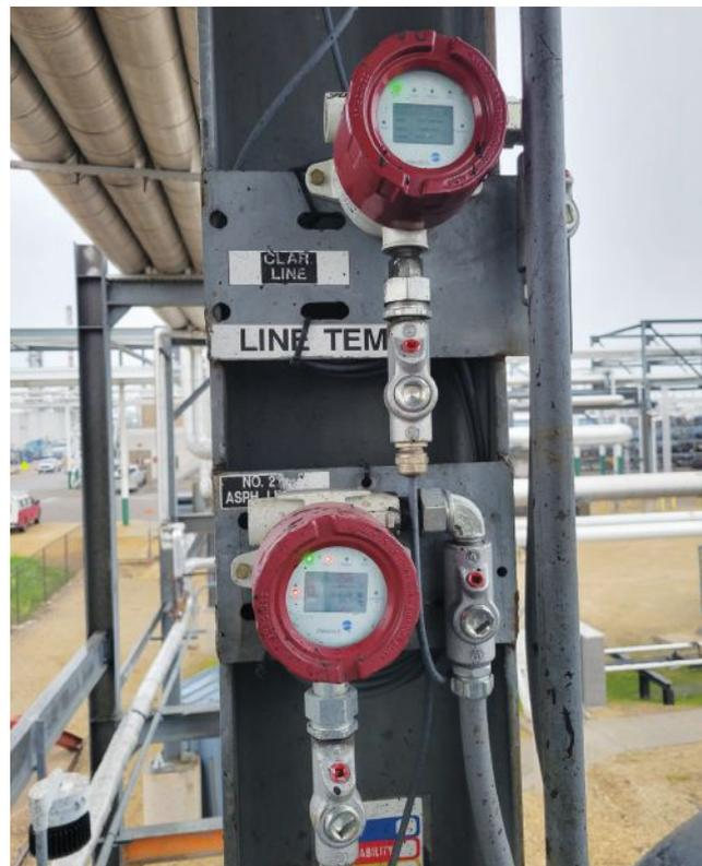
Figure 4: SME-TRD transmitter displaying real-time viscosity readings from SRV deployed at an asphalt terminal
